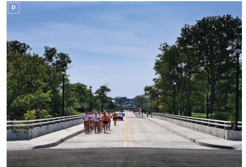
U.S. Department of Navy D Street Bridge GREAT LAKES NAVAL STATION, ILLINOIS
