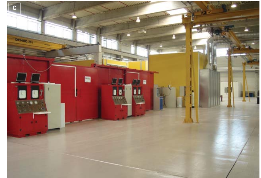
Cameron International Manufacturing Facility & Office PLOIESTI, ROMANIA
