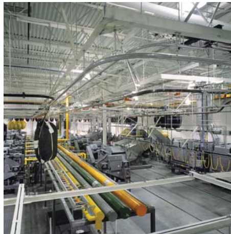
ARAMARK UNIFORM SERVICES Chicago, Illinois 161,000 square foot, laundry processing facility
