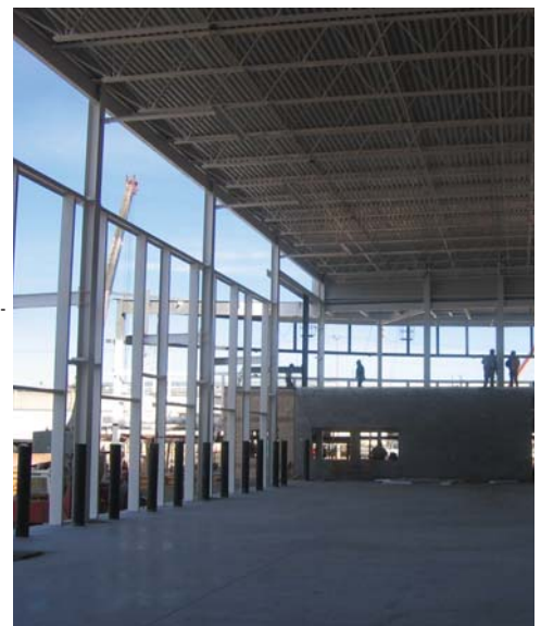
CONSTRUCTION SHOTS OF FRUGASA Chihuahua, Mexico February 2006
