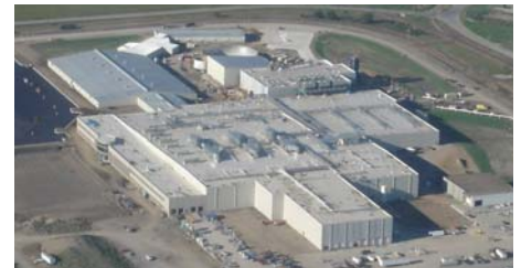
TRIUMPH FOODS LLC St. Joseph, Missouri 625,000 square foot, $130 M pork processing facility
