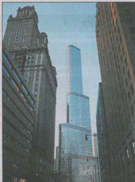
The Trump Hotel & Tower has a luminous facade. E. JASON WAMBSGANS/TRIBUNE PHOTO
